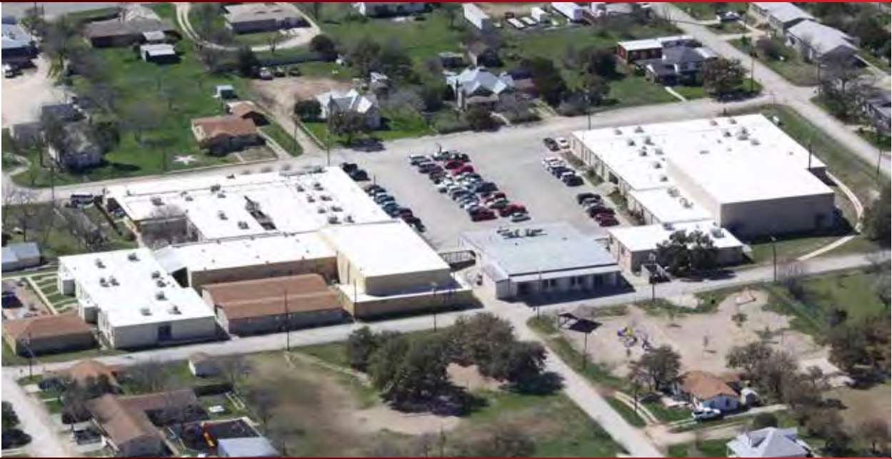
Jarrell ISD - Installed in 2018
