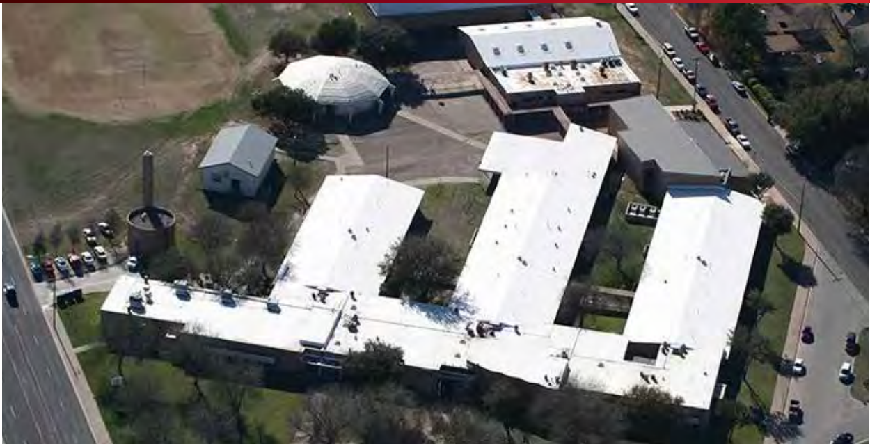
Waco ISD - Sul Ross Elementary - Installed in 2010
