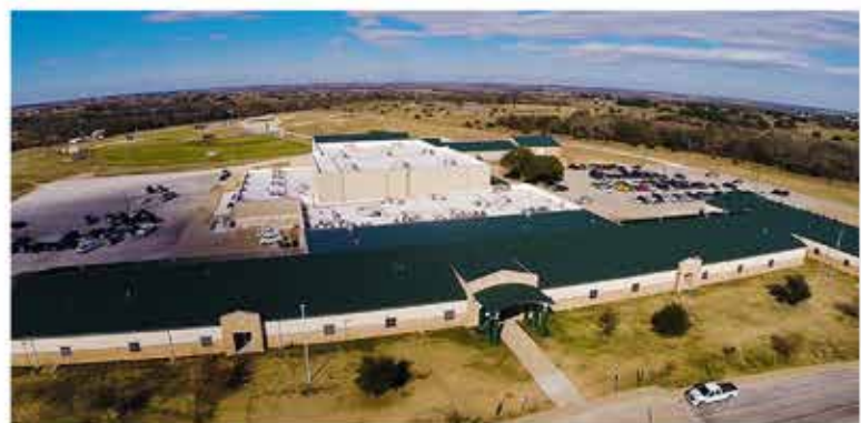
Dublin ISD - Installed in 2015
