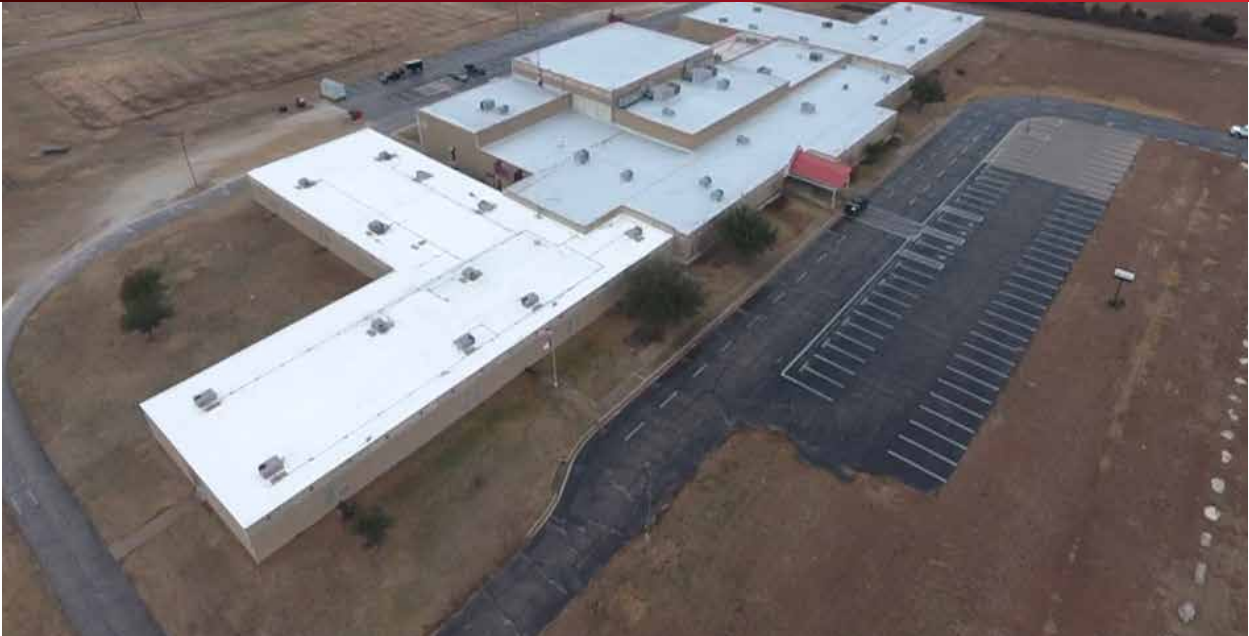
Lorena ISD - Lorena Elementary School - Installed in 2017
