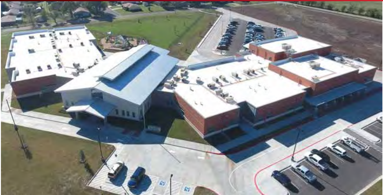
Clifton ISD High School - Installed in 2018
