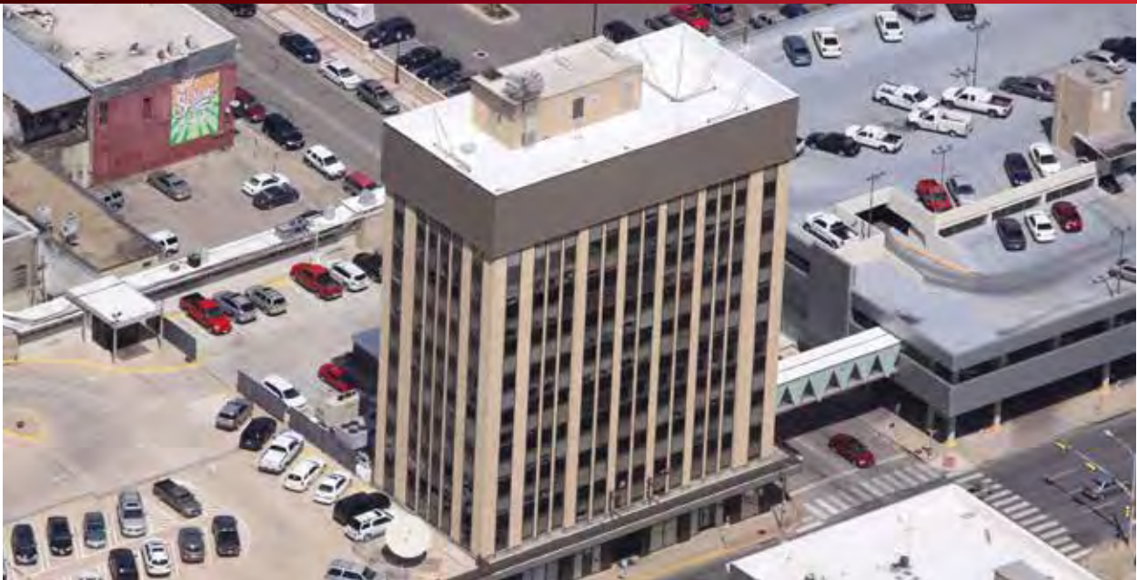
Waco ISD - A.J. Moore Academy - Installed in 2006
