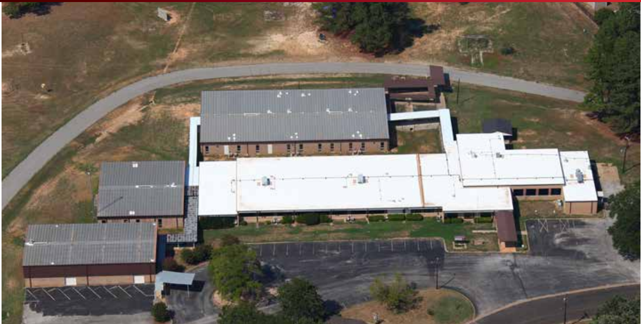
Henderson ISD Northside Elementary - Installed in 2011
