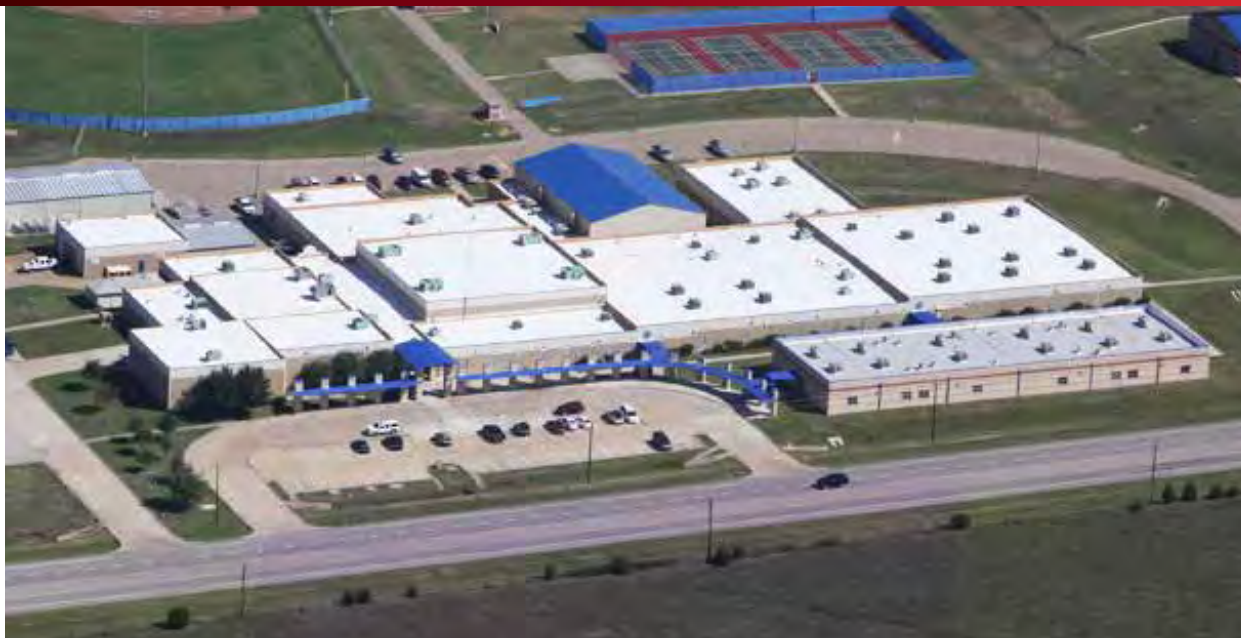
Clifton ISD Intermediate - Installed in 2007
