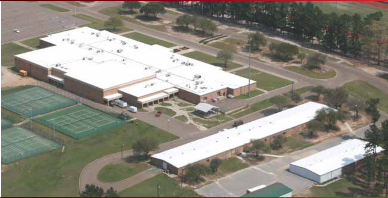
Avery ISD - Installed in 2012
