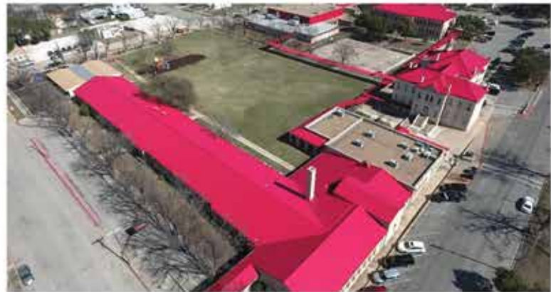
Sonora ISD - Installed in 2017
