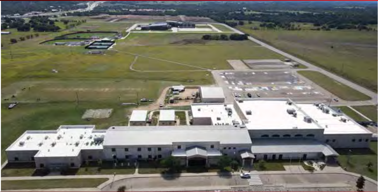
Troy ISD High School - Installed in 2020
