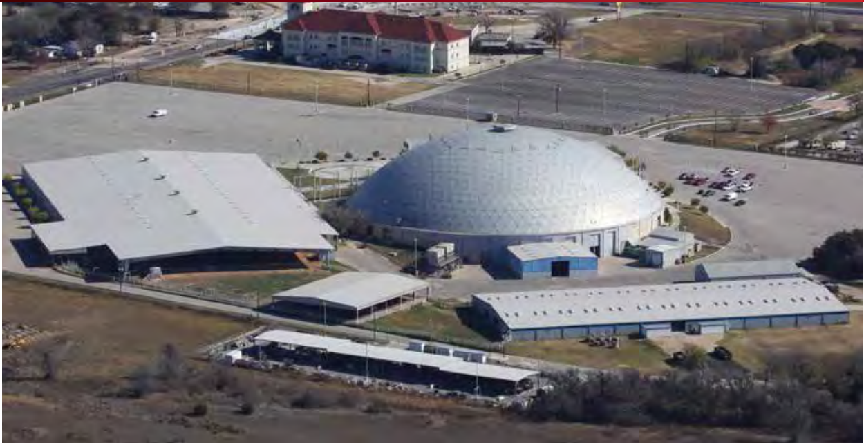
Cameron County Detention Center - Installed in 2008
