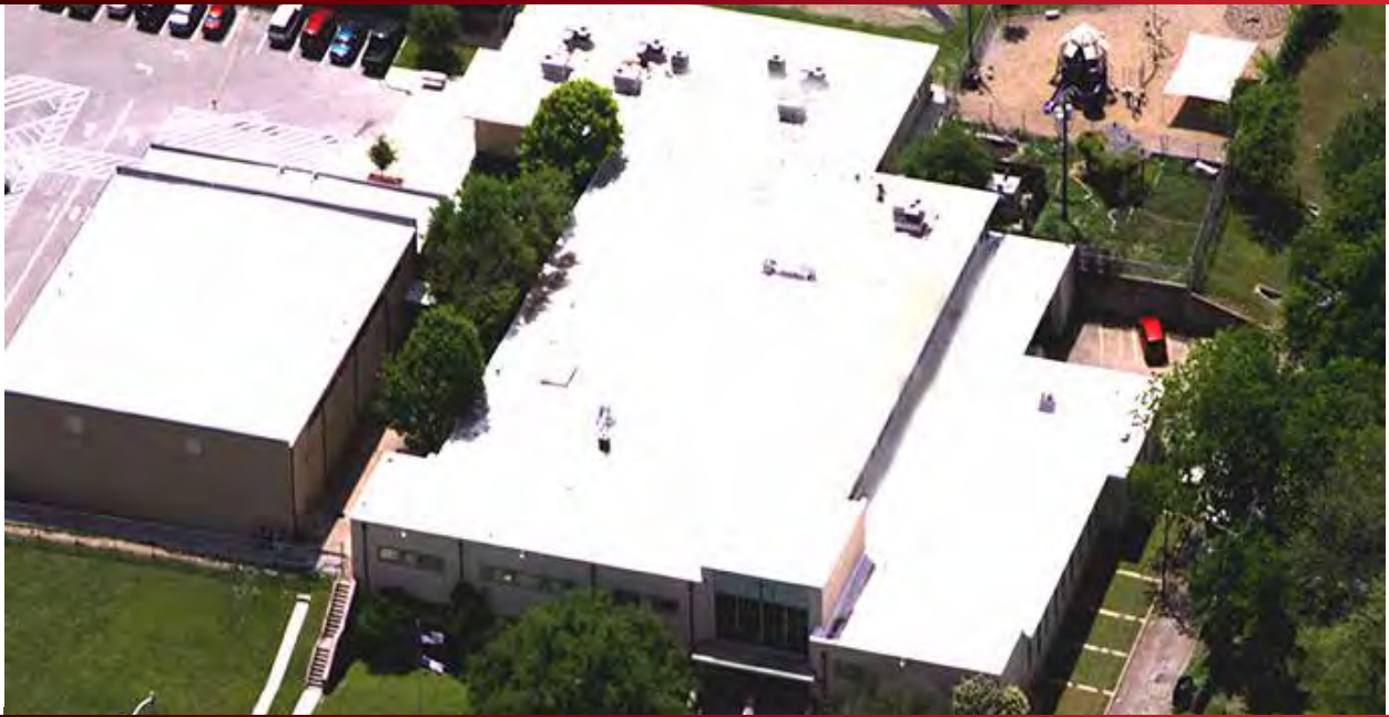
Bruceville - Eddy ISD - Installed in 2003
