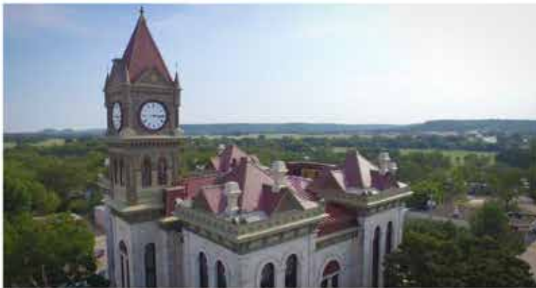
Bosque County Courthouse - Installed in 2014
