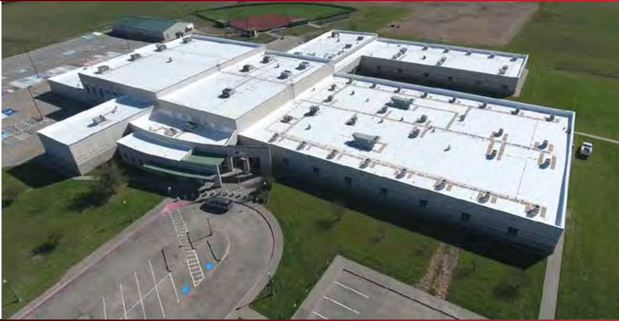
Commerce ISD - Installed in 2019
