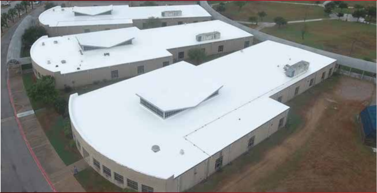
San Benito ISD - Fred Booth Elementary Annex - Installed in 2018
