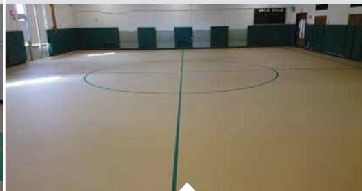
HILLSIDE ELEMENTARY SCHOOL Hastings-on-Hudson, NY Installed in 2016
