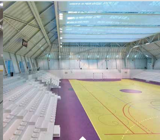
PALAIS DES SPORTS Loudeac, France Installed in 2014
