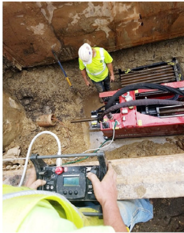
Enhanced safety. Some modern pulling machine designs free the operator from the pit, offering a superior view of the operation and of worksite surroundings during an installation
