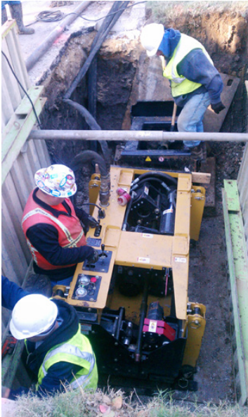
Machine pit dimensions need to be only big enough to accommodate a 4-foot by 12-foot shore box, at a depth not much deeper than the lay of pipe being replaced
