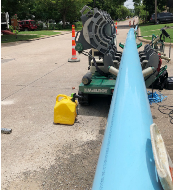
Joint fusing and pipe staging area. Sticks of PVC are joined to full run length prior to the day of the burst, stored conveniently out of the way near the insertion point
