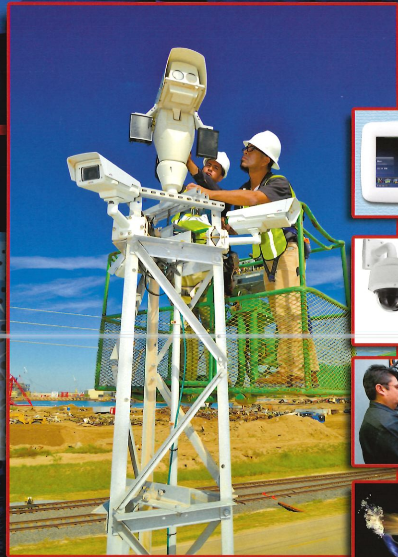
American Surveillance crews servicing video surveillance cameras on a 30-ft Systems tower at the Port of Brownsville.
