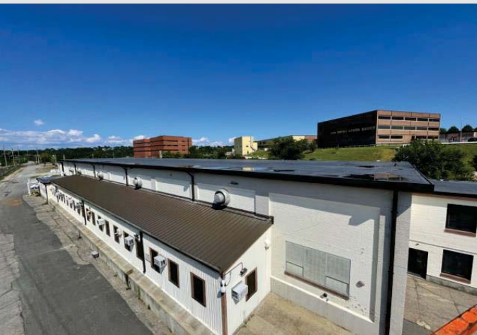
EPDM/Standing Seam Metal/Gutters Newport, RI
