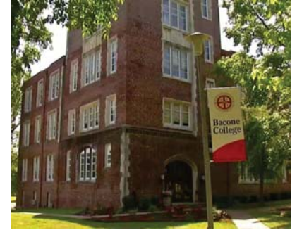
Bacone College: Upgrade of HVAC systems with ClimateMaster, and Air Side Products(ASP) and upgrading building temperature control from antiquated thermostats to the Cloud.
