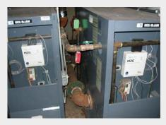
These ALM controllers do not require calibration. They infer boiler temperature settings and are compatible with OTR systems.
