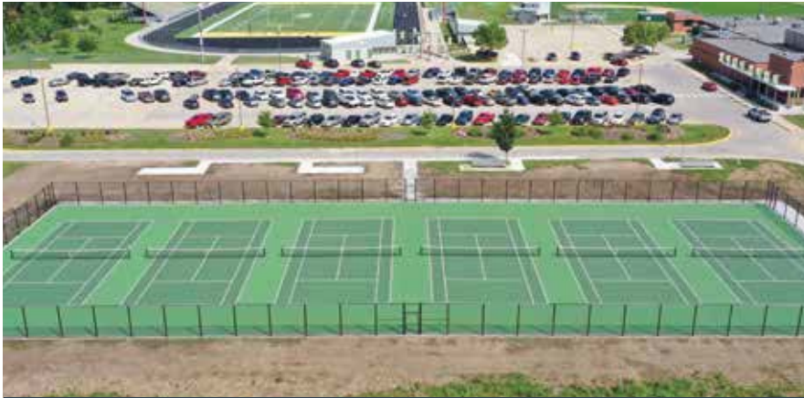
Des Moines, IA - Saydel Community School District - Tennis Facility
