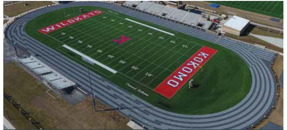
Kokomo, IN - Walter Cross Track
