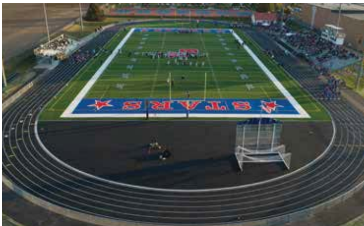
Thorntown, IN - Western Boone Track & Field
