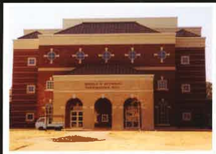
Reynolds Performance Hall - UCA Metal Roof
