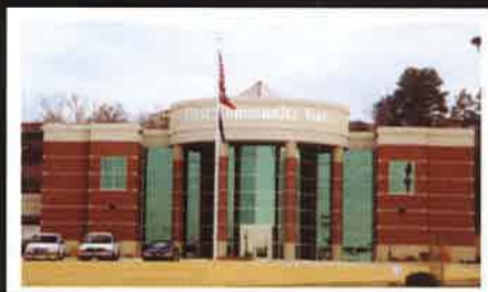
First Community Bank - Hwy. 64 W Flat Roof
