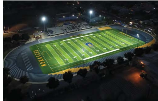
Installation at Exeter Union High School, Exeter, CA.
